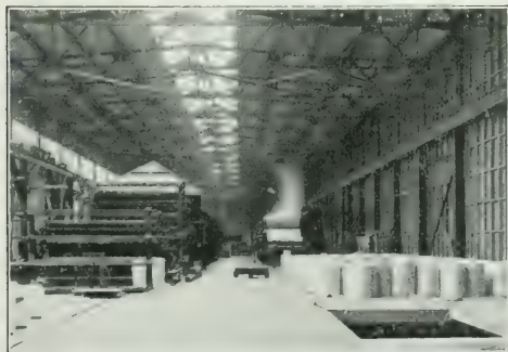
MACHINE ROOM BATHURST LUMBER CO.
